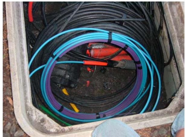
Figure 8. Installed additional tube and cable
