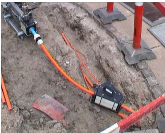
Figure 10. Additional jetting Copenhagen
