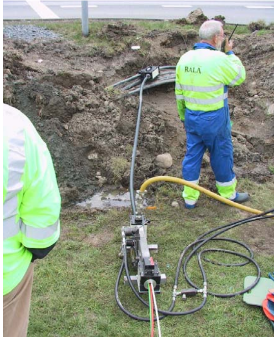
Figure 9. Additional jetting of 3 tubes of 10 mm
