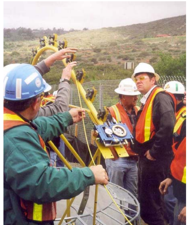
Figure 5. Jetting micro-cables with buffering
